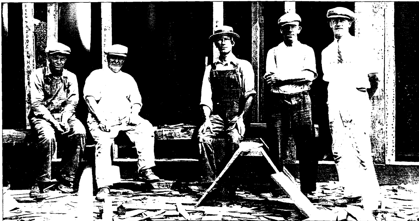
Men on the job/1927-28 restoration. Left to right: Fletcher Ross; Arthur Williams, mason; William King; Archibald Cartwright, carpenter and builder; and (unidentified), are standing before the west end of the south wall. Note the replacement studs behind them salvaged from the Paddock House and marked Paddock. Photo: SPNEA collection
